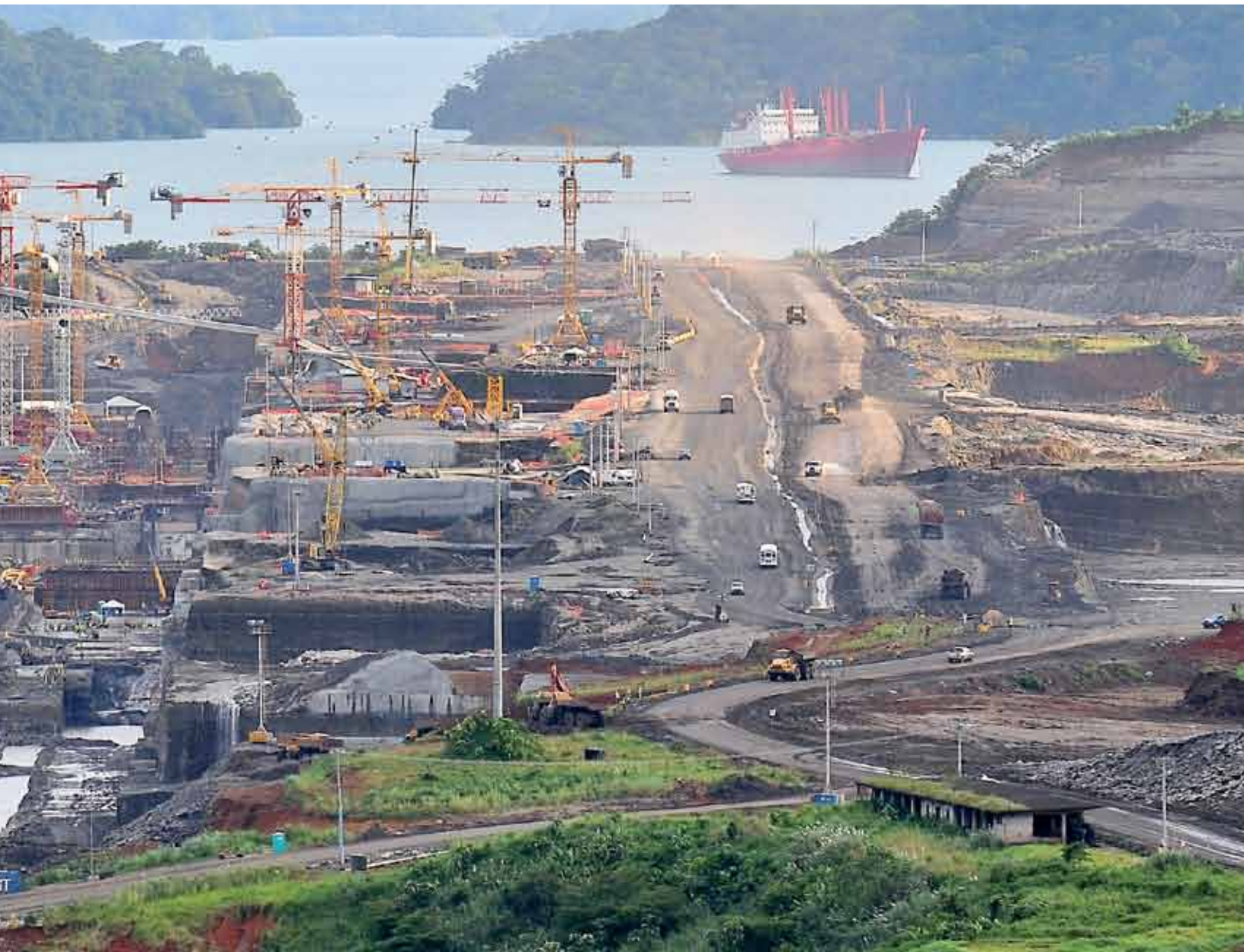
Construction of the Third Set of Locks on the Atlantic Side is under way at the former 1939 US excavation site. Progress of the excavation gave way to civil works which started in July 2011 with the placement of the first batch of structural concrete on the floor of the upper chamber.
