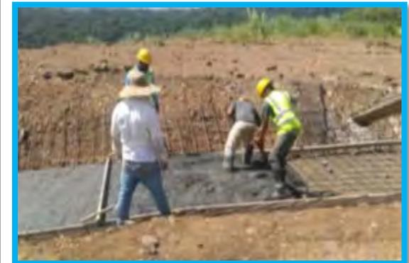
**Picture N 48:** PS-6 Subcontractor Avantis continues working in the drop structure construction. Concrete pouring is being executed in the upper parts of this disposal – SCP Measures 32-34
