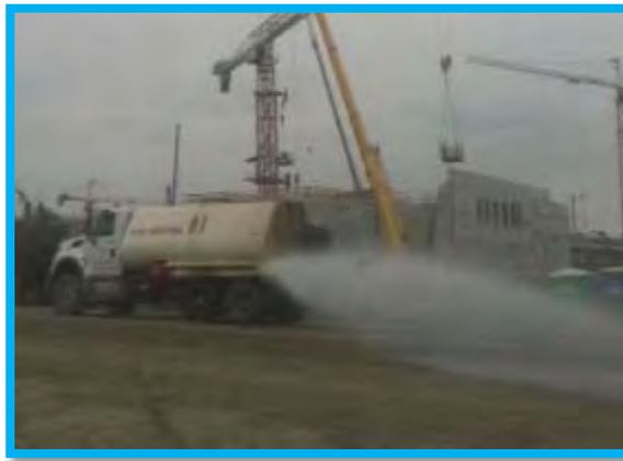
**Picture N°8:** PS-2-4 Moistening of roads to reduce the generation of dust continues. Trucks sprinkle water through the roads and minimize the dust
