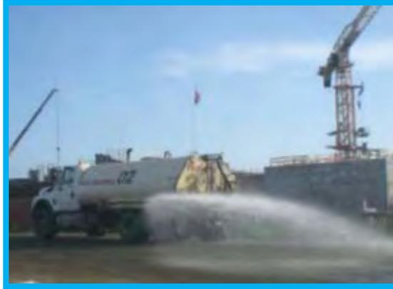
**Picture N 20:** PS-2-4 Moistening of roads in front of the warehouse was observed several times. This measure helps to reduce the generation of dust – SCP Measures 32-34
