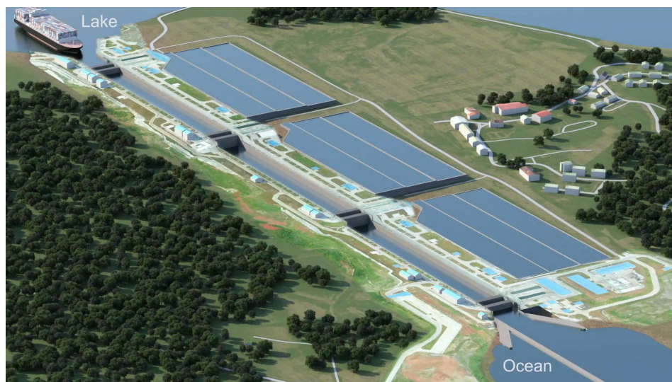
Figure 3-4: Agua Clara Neopanamax Water Savings Basins
