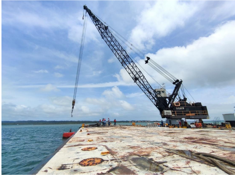
Figure 5 Installation and removal of mooring buoys
