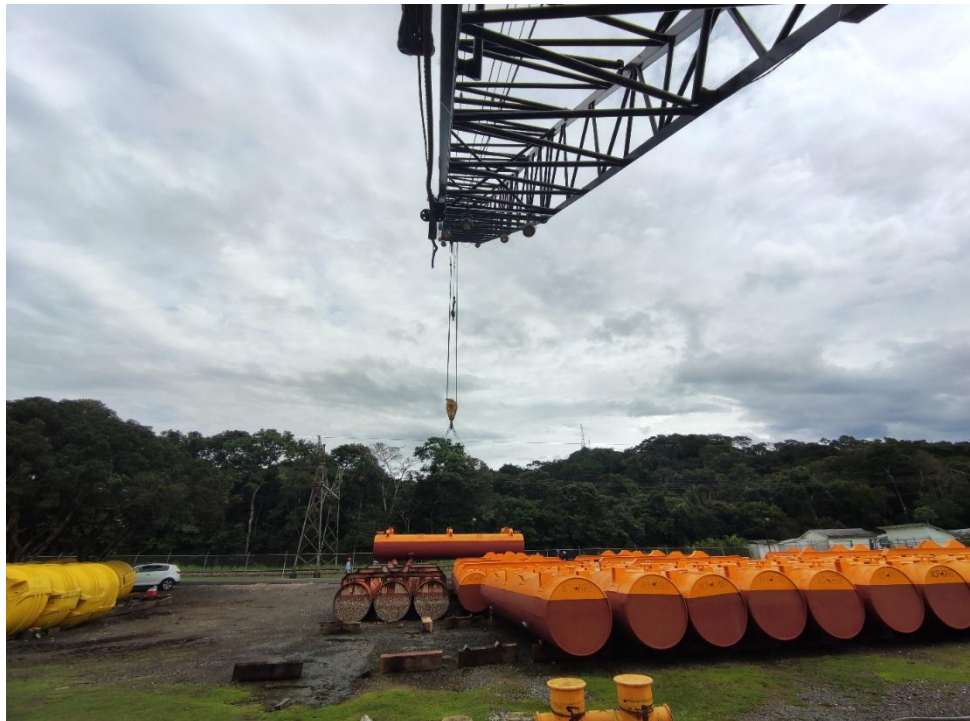
Figure 6 Pontoon lifting operations for Quibián dredger pipeline support
