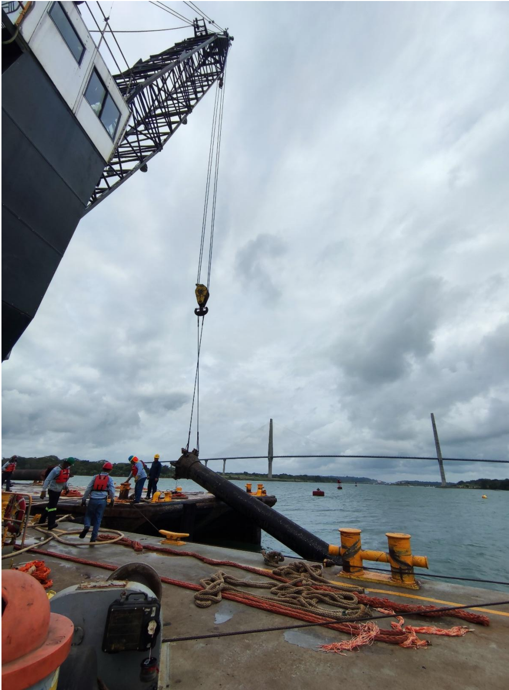
Figure 7 Pipeline hoisting procedures for the Quibián dredger
